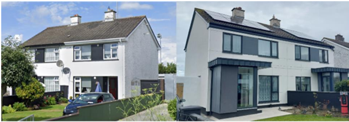
Figure 2: Showing (RHS) pre works elevation with (LHS) completed modular retrofit.
